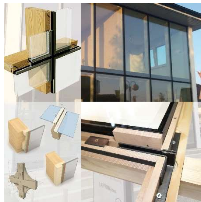
Figure 1. Applications of multi-story timber-glass facades, Blaue Lagune HAAS Haus, Austria (top right) and various developed connection
