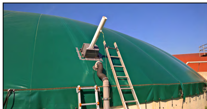
Figure 1: Measurement of the methane diffusion rate from an air-inflated double membrane dome.
